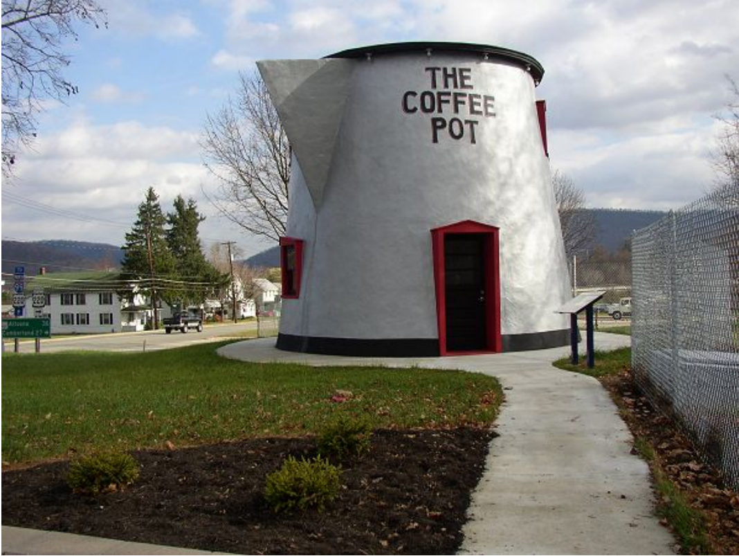
Coffee Pot Building just west of Bedford, PA on the Lincoln Highway Photo by Ron Johnson
